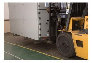
Figure 5: Lifting of switchgear frames with forklift
