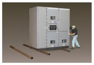
Figure 7: Movement of the frames with rollers.
