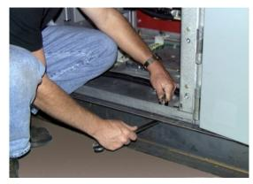
Figure 10: Unbolting the shipping bases.
