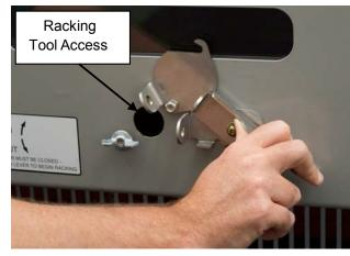
Figure 24: Racking release handle
