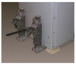
Figure 11: Using jacks to lower the frames onto wood blocks.
