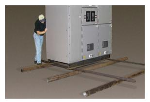
Figure 9: Lateral movement of the frames with rollers.
