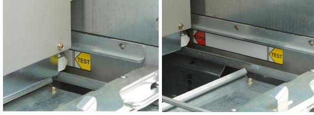
Figure 26:(a): Circuit breaker in TEST position
