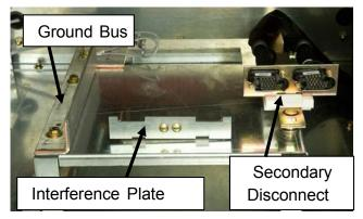
Figure 31: Circuit breaker self-aligning secondaries
