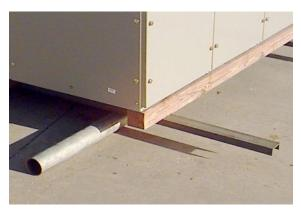
Figure 8: Position rails as shown for lateral movement.
