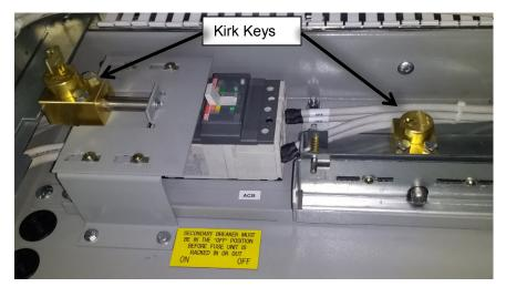
Figure 28: Secondary breaker interlock in 'ON' position and Blocking mechanism withdrawn position.
