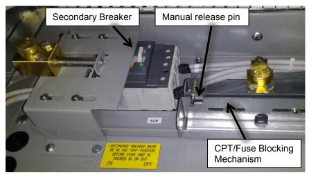
Figure 27: Secondary Breaker in 'OFF' position and Blocking mechanism withdrawn position using the Kirk Key.
