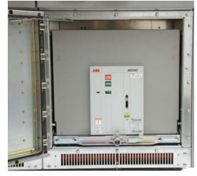
Figure 23: Circuit breaker in DISCONNECT position
