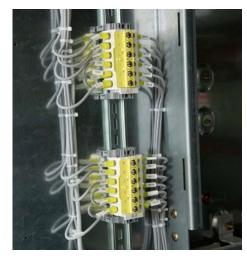
Figure 13: Current Transformer Shorting Blocks.
