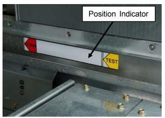
Figure 25: Circuit breaker position indicator
