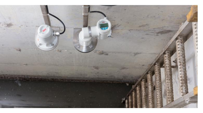
01 ABB laser level transmitters used in municipal wells to measure wastewater level. Lasers enable level monitoring measurement for various dry bulk solids and liquids stored in vessels. They can measure through narrow gaps and down to the bottom of vessels. They work in all types of storage vessels, including silos, tanks, feed chutes, bunkers, and hoppers.
