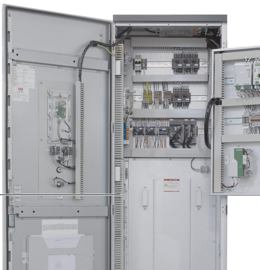
Duct for auxiliary and control cables (1)
