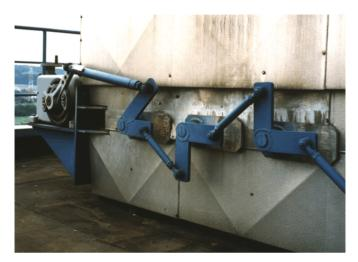
Figure 33: Controlling exhaust gas using a rotary actuator on a multi-leaf valve
