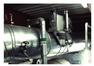
Figure 36: Rotary actuator (air control)
