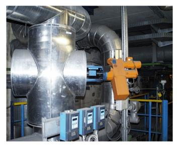
Figure 35: Horizontally installed linear actuator (air control)
