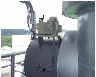
Figure 37: Milling air control; rotary actuator RHD250 (rated torque 250 Nm)
