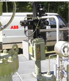
Commissioning support from specialist ABB personnel during installation of an explosion-Change from one to two columns proof linear actuator RSDE10
