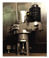
Figure 34: Linear actuator (feed-water preheating)
