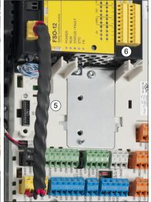
7. Connect the power supply wires to the FSO terminal X112. Use the tightening torque of 0.24 Nm (2.1 lbf·in) for the FSO terminals. Use proper cable strain relief. See also section *Power supply connection/cables* on page 203.
