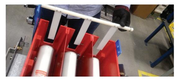
13 Tighten the plastic bolts on the cover that supports the blown fuse switch.
