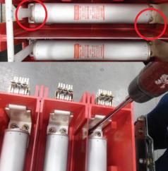
— 08 Extract the insulation barrier between the fuses.
