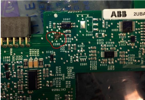
Figure 15: Q603 burned on control board
