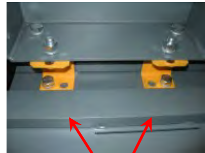
(2) Cleats at Belt / Pulley Housing
