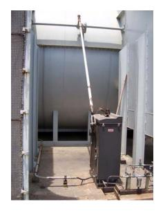
Typical installation of LP Type Linear Pneumatic Actuator on Boiler Over fire Air control.
