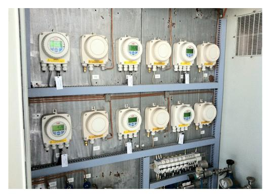
Endura AZ20 combustion gas analyzers in situ
