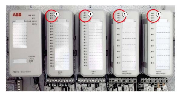
Figure 10-5 Example of S800 I/O station
