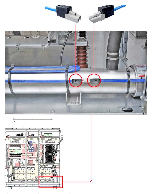
Figure 5-14 Heating cable connection
