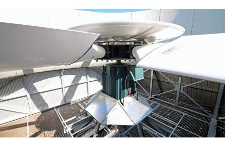
Cooling towers are used in food processing plants all over the world. Maintenance and failure of the gearbox, and associated components, is often problematic with traditional systems. The Baldor-Reliance® RPM AC direct drive cooling tower elminates these problems by coupling the motor directed to the fan and controlling it with a unique drive.
