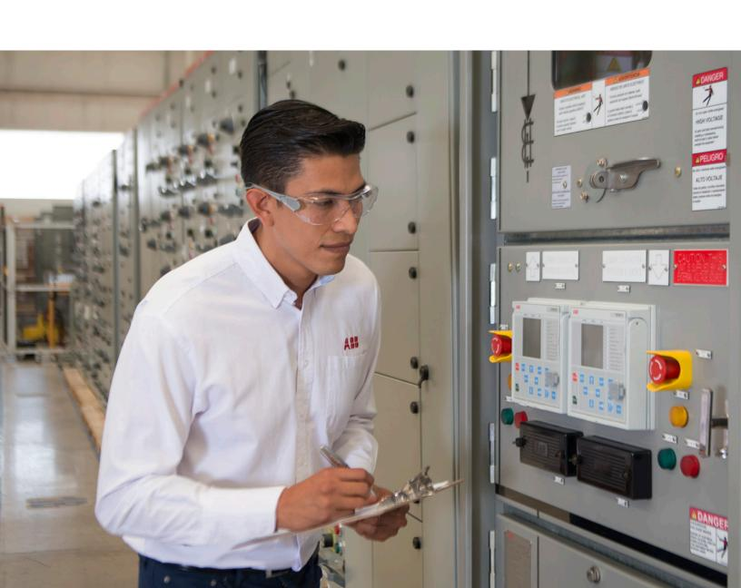
SafeGear® Motor Control Center Controller
